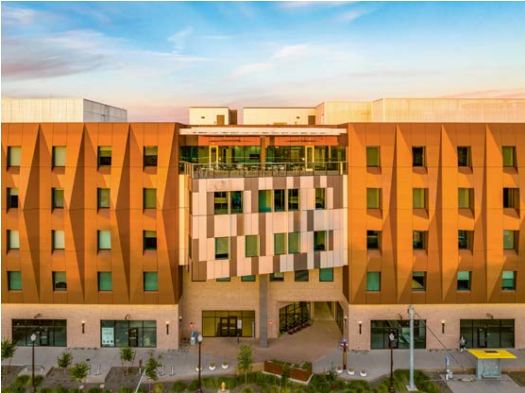
▼ Arizona State University, Tempe, Arizona, USA, ALUCOBOND® PLUS
